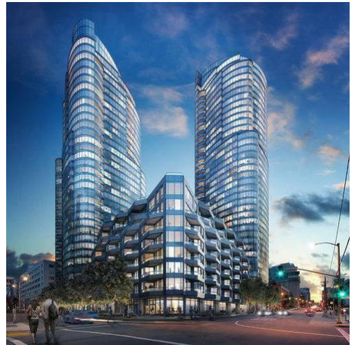
The project features two towers that rise 42 and 37-stories and two plaza buildings of eight stories each, connected by a shared podium.
